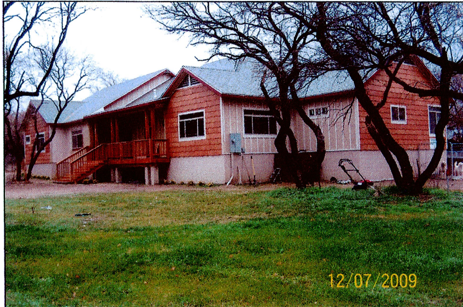
FRONT VIEW (from right front corner)
