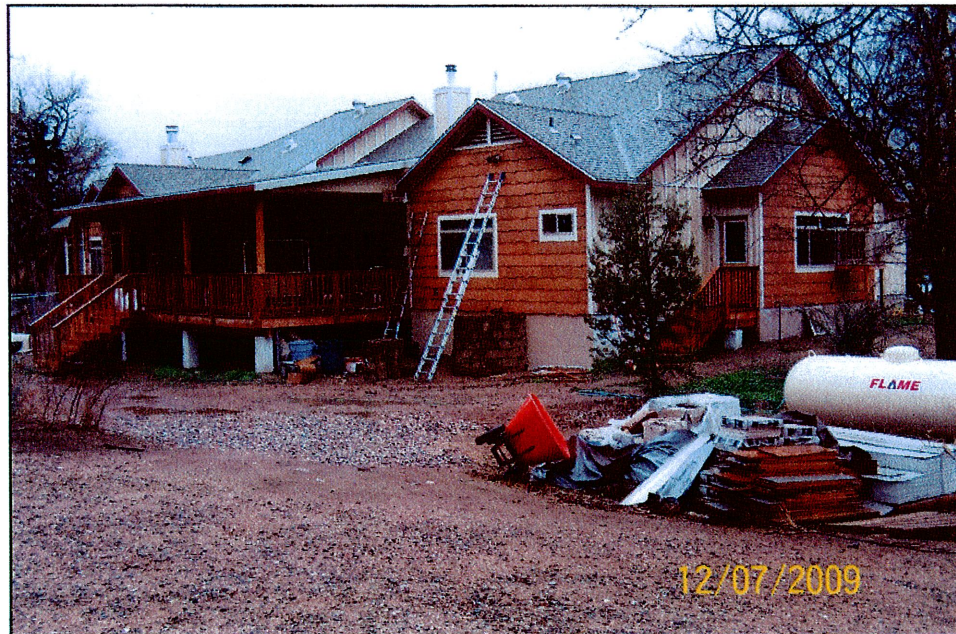
REAR VIEW (from left rear corner)
