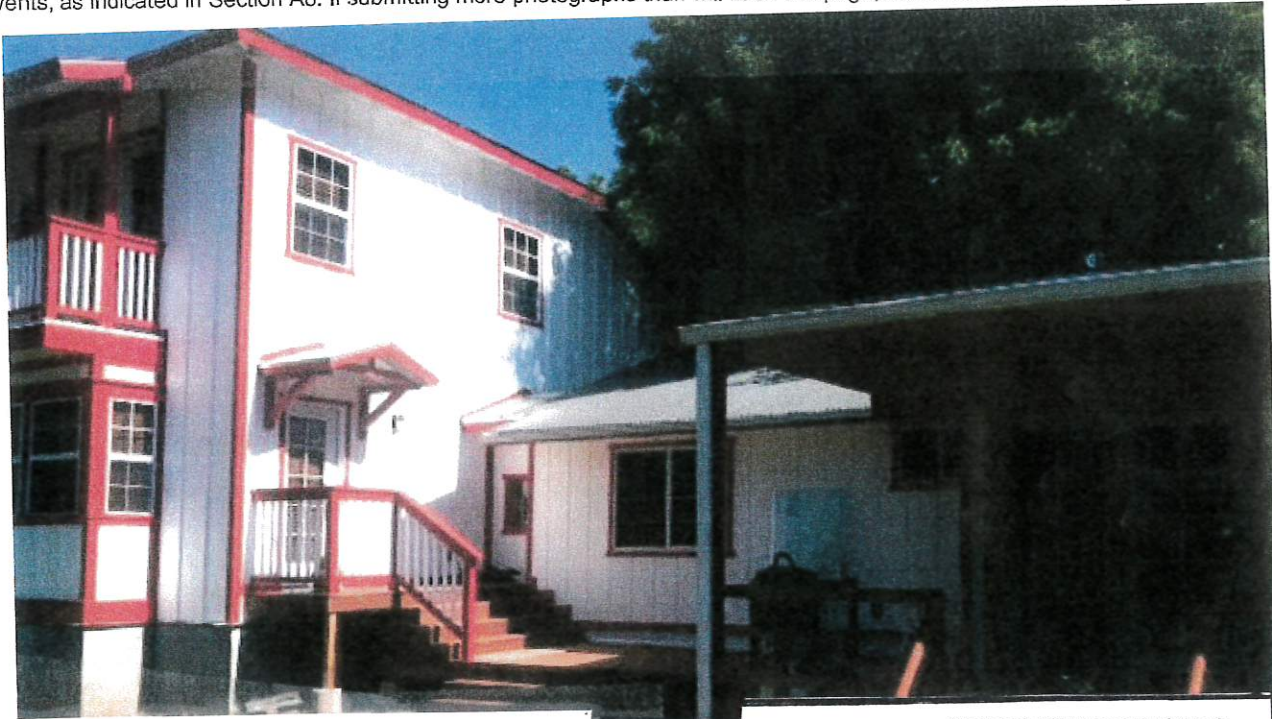
PHOTO #1, S.E. CORNER OF ADDITION TO LEFT OF ORIGINAL HOUSE
