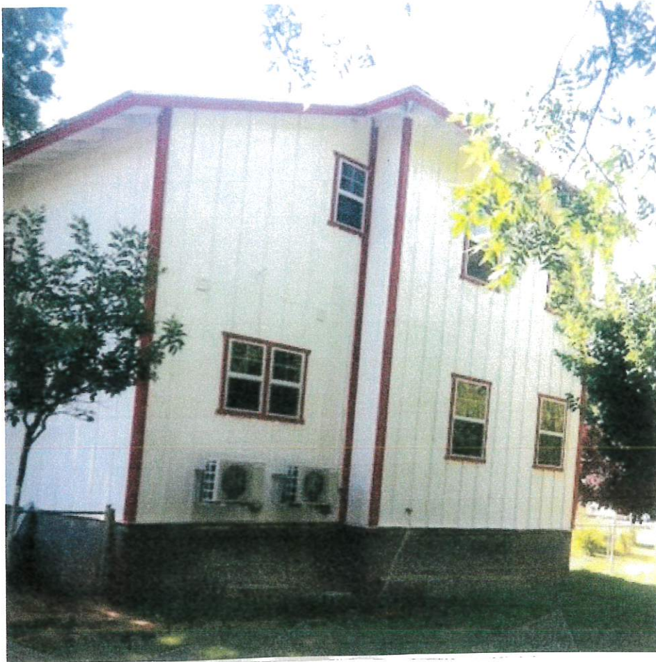
PHOTO #5 , LOOKING S.E. AT WEST SIDE OF ADDITION. PLEASE NOTE AIR CONDITIONER PAIR ESTABLISHED ABOVE FIRST FLOOR. THREE OF THE FLOW OUTLETS ARE PRESENT JUST ABOVE GROUND LEVEL (BUT DIFFICULT TO SEE IN SHADED AREAS)
