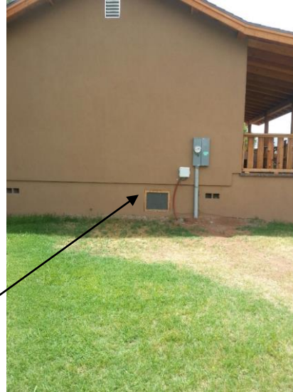
Side View (with flood vent) North side of house
