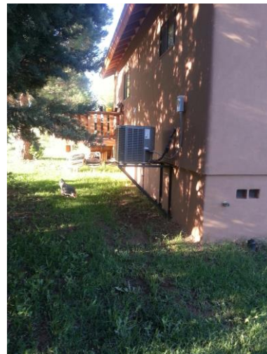
Back View (showing Air Conditioner Compressor) East Side of House
