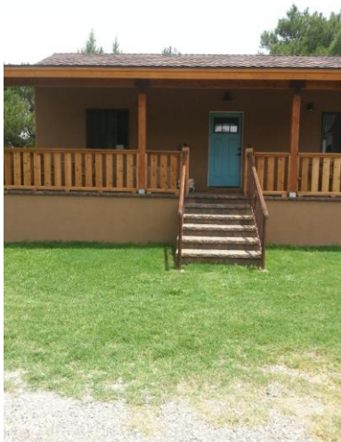
Front View West Side of House
