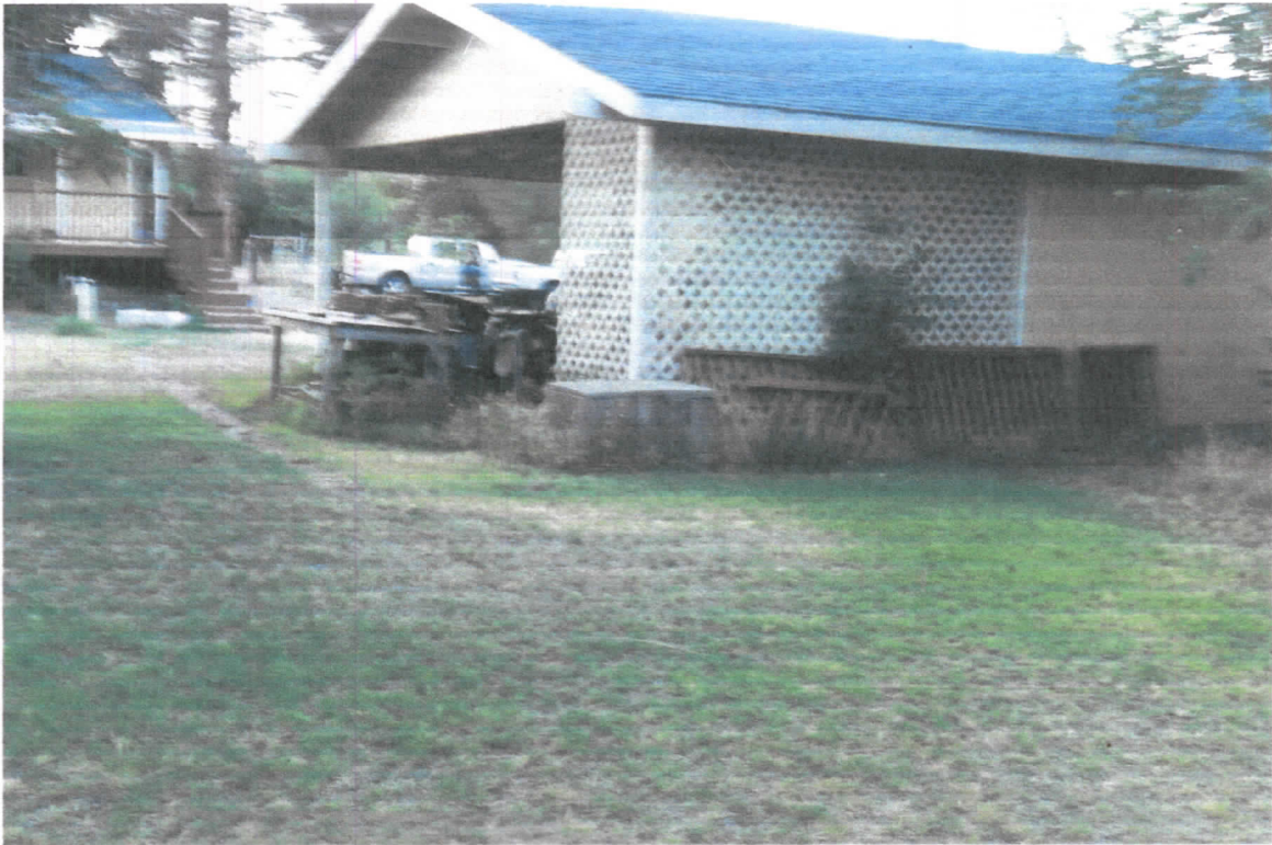
LOOKING E.E.S. BLDG. WITH ELECT. POWER
