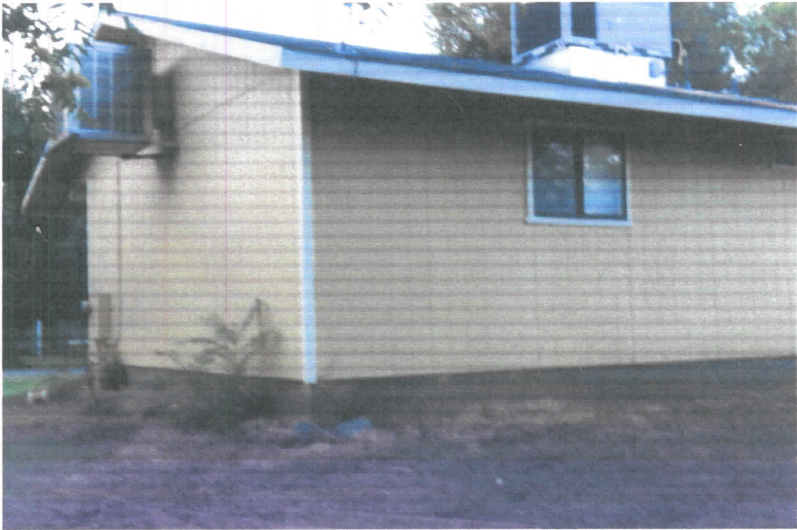
N.W. CORNER HOUSE, AIR CONDITIONER
