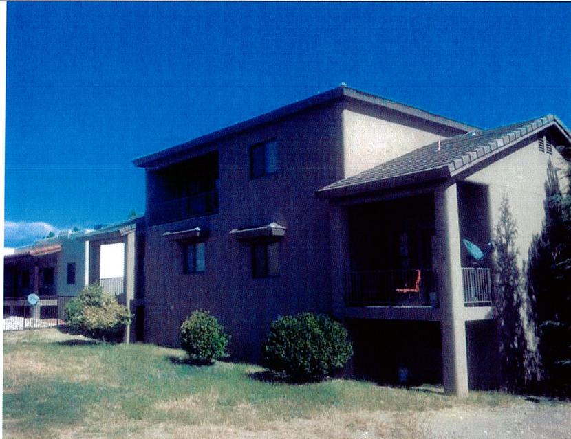
West face of building 10/28/2013
