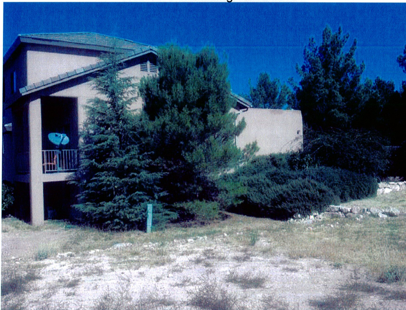
South face of Building 10/28/2013
