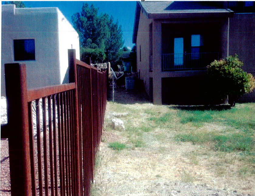
North face of Building 10/28/2013
