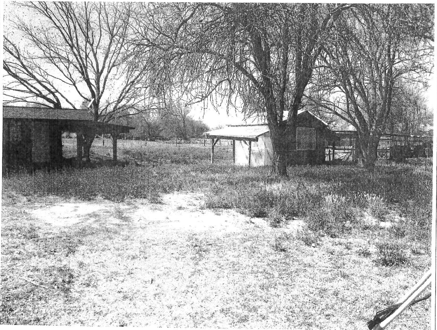
Side/rear of greenhouse 03/28/2014
