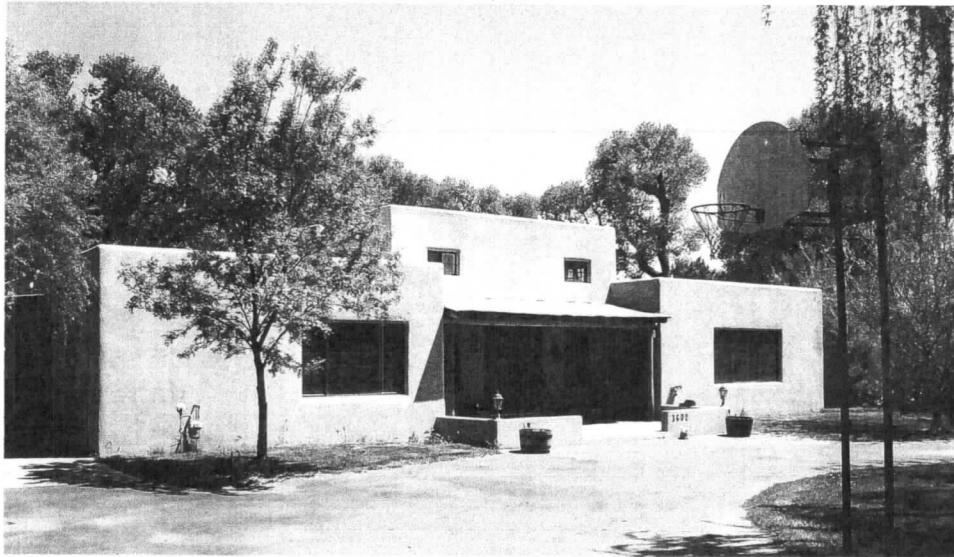
HOUSE FRONT (TAKEN 4/19/06)
