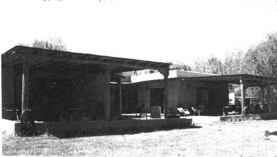
HOUSE REAR (TAKEN 4/19/06)
