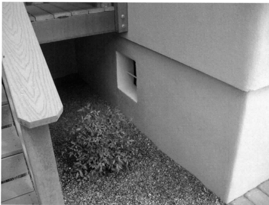
10/07/2009 Left Side (west flood opening by entrance)
