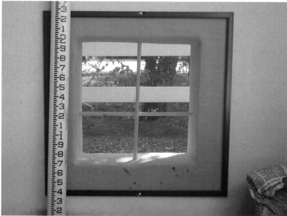
10/07/2009 Inside view (southeast flood opening)
