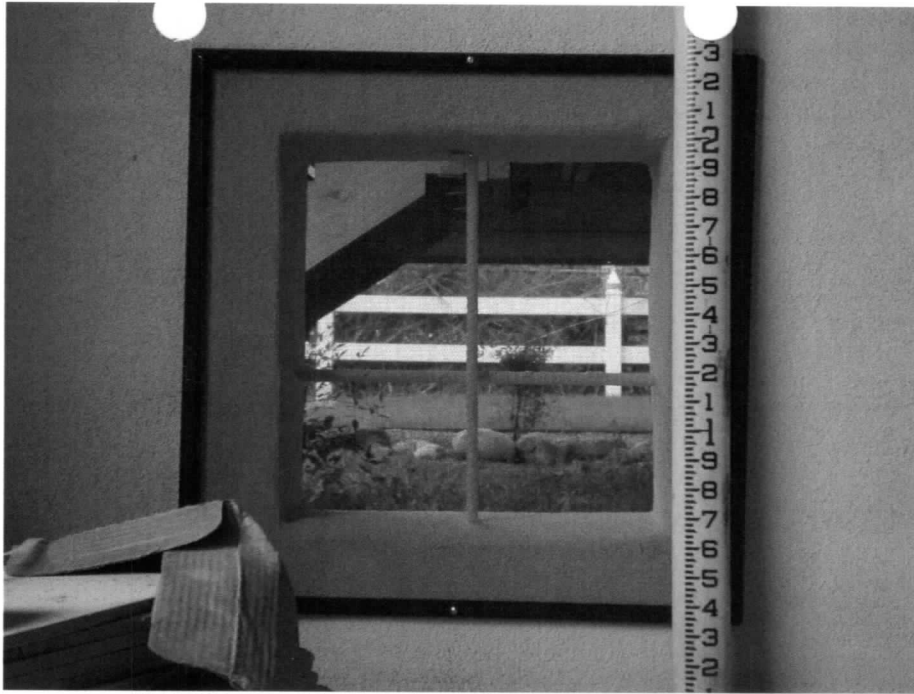
10/07/2009 Inside view (west flood opening by entrance)
