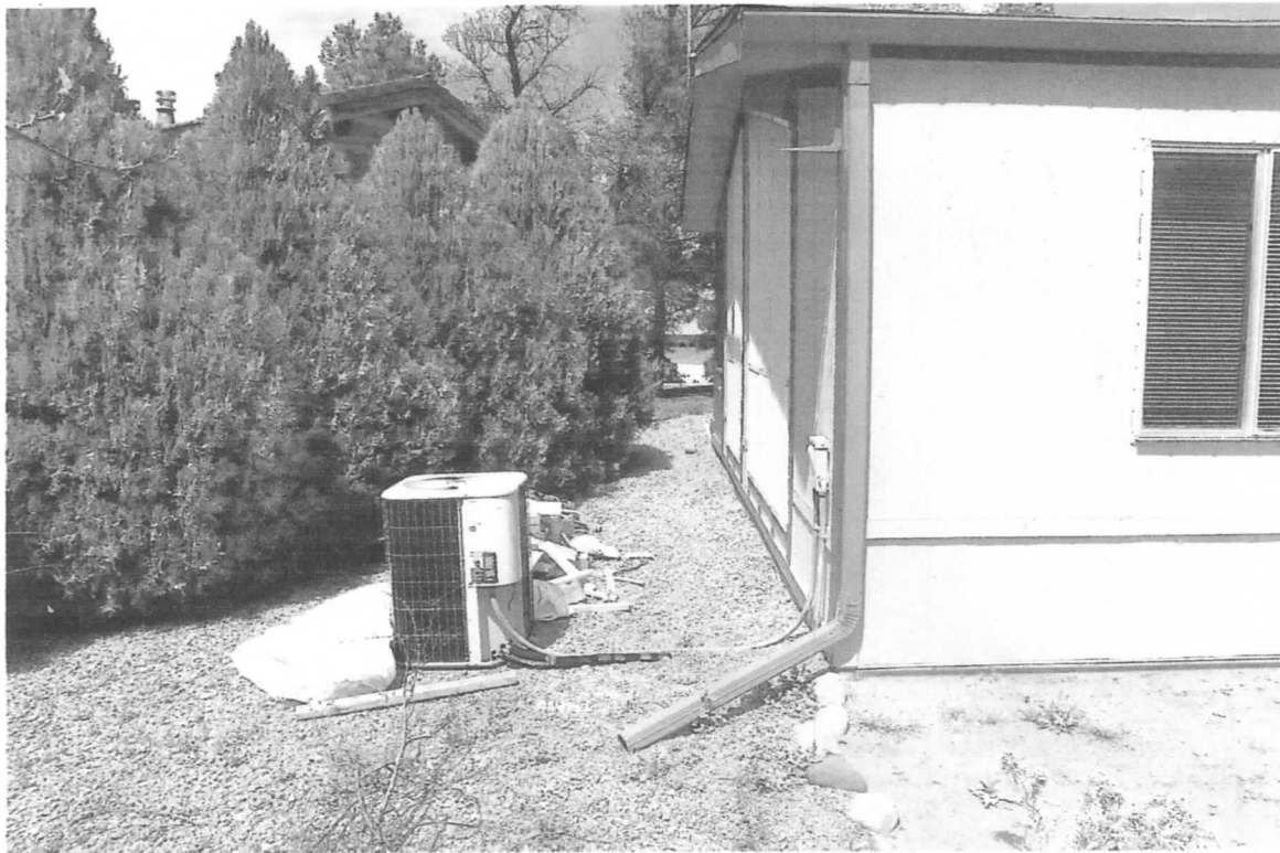
S.W. CORNER OF BUILDING
