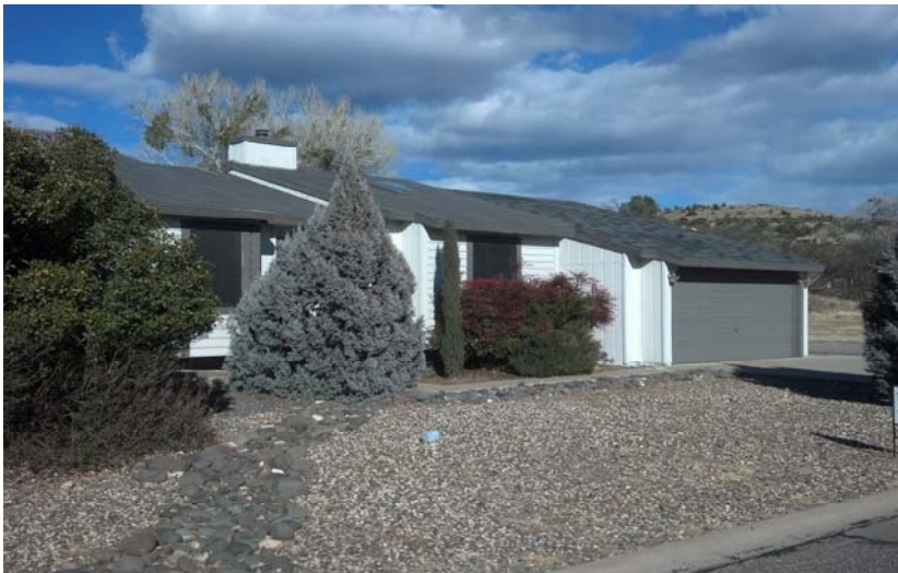
SE FACE OF BUILDING
