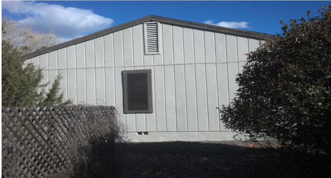
EAST FACE OF BUILDING
