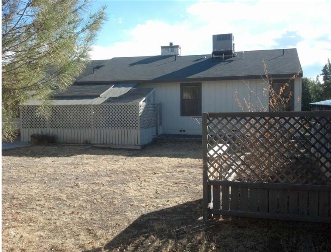
NORTH FACE OF BUILDING
