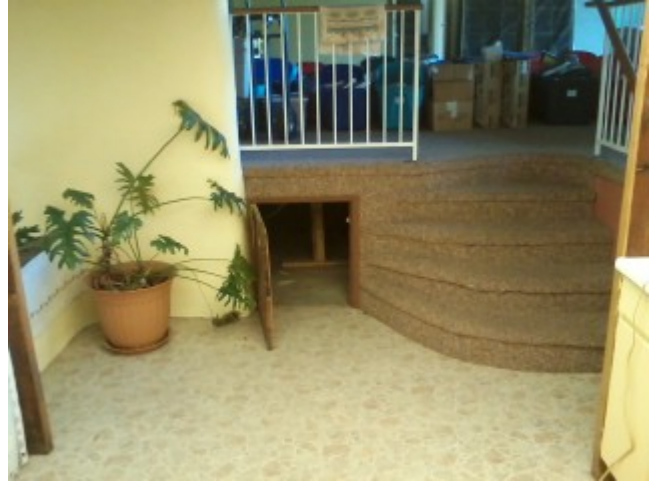
PARTIAL BASEMENT, STORAGE OPENING, AND UPPER MAIN FLOOR
