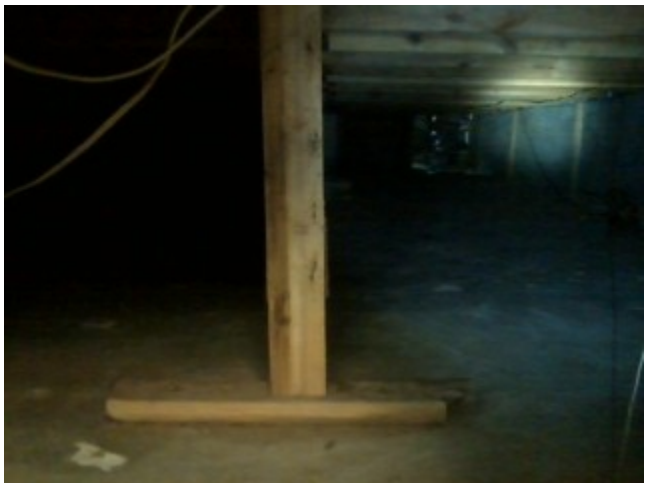
LOWER STORAGE AREA. SAME LEVEL AS BASEMENT
