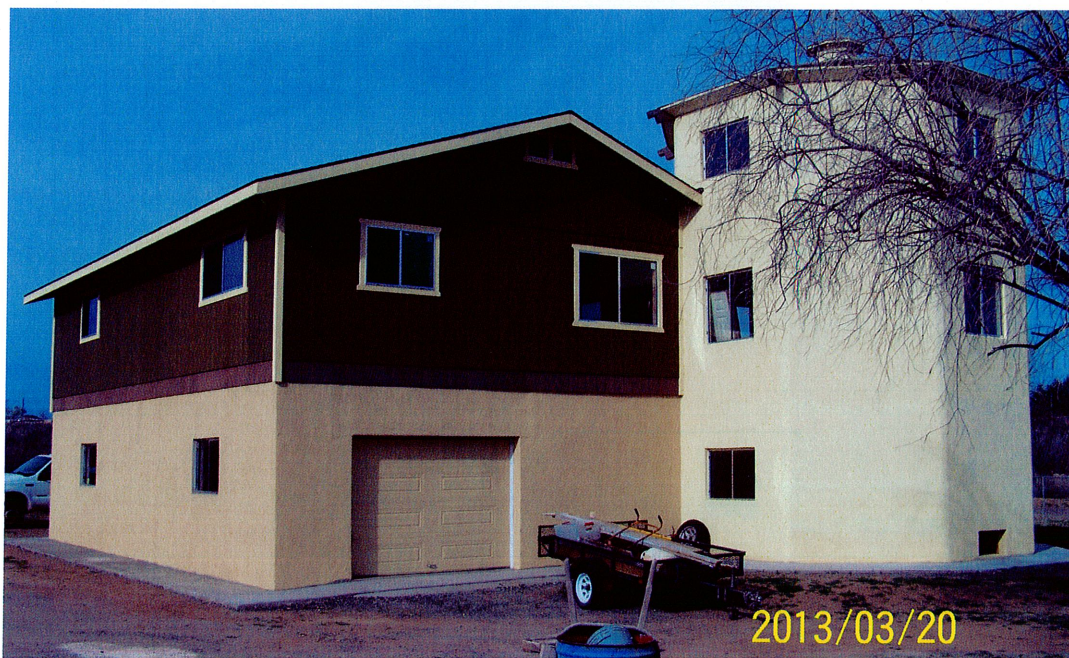
Back view, from left rear corner.
