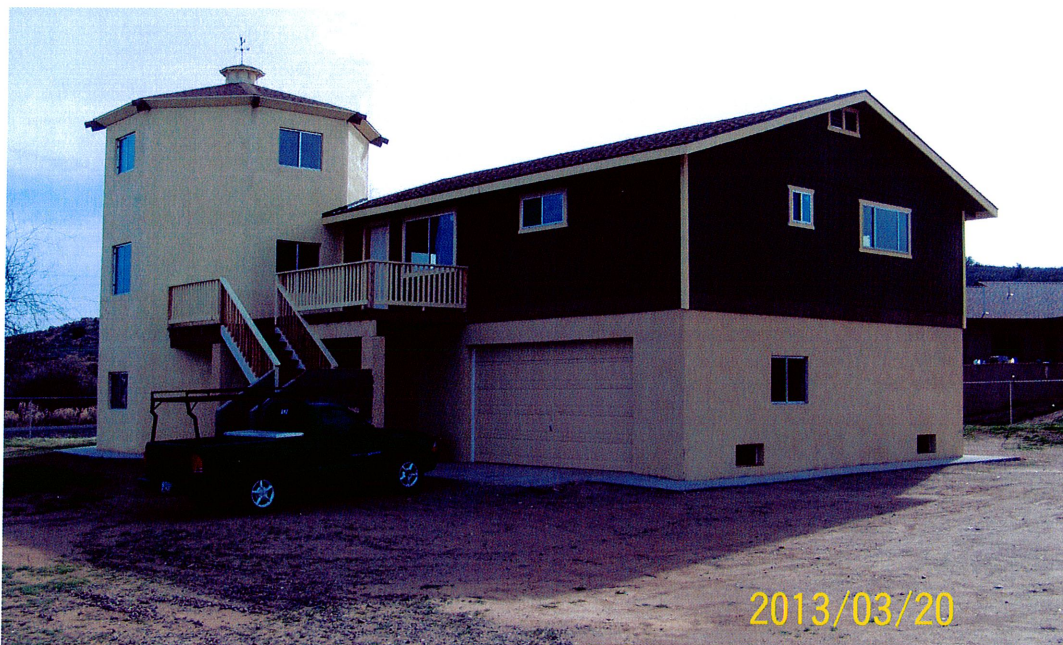
Front view, from front right corner.
