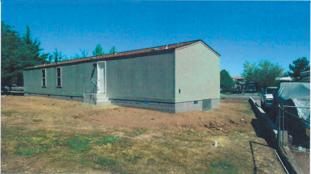
Photo Two Caption BACK AND EAST END LOOKING NORTH TOWARDS STREET 4-6-17
