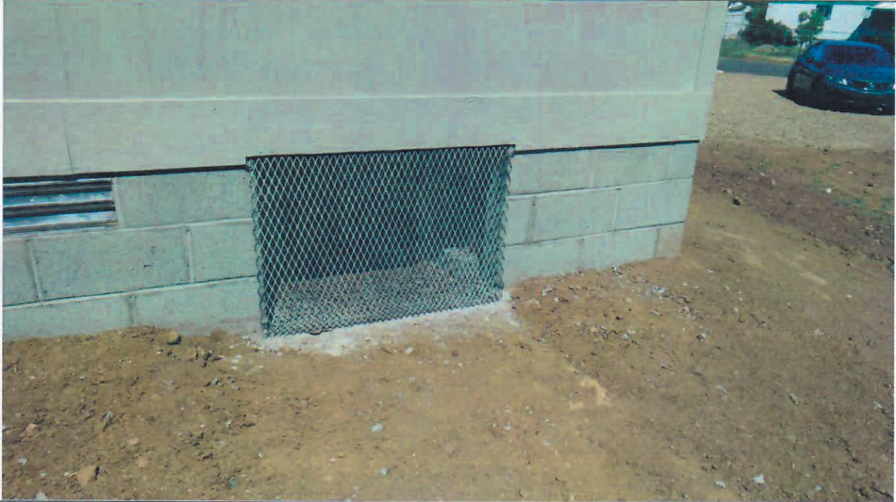
Photo One Caption EAST END CRAWLSPACE ACCESS SCREEN 04-06-17
