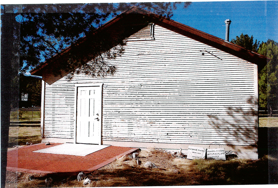
South View Entrance 10/20/14
