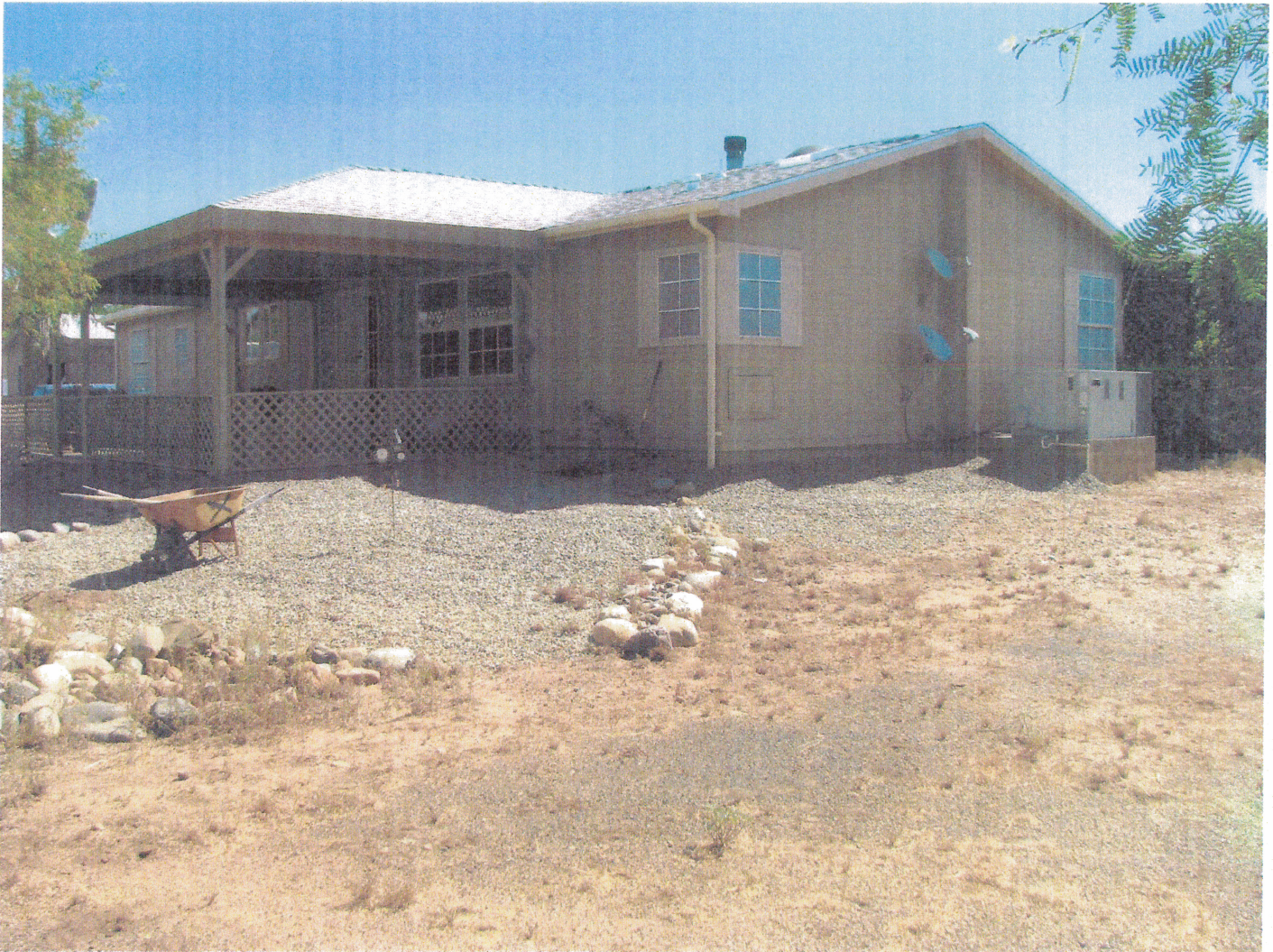
SOUTH END/WEST SIDE - C2E ON A/C PAD 06-27-2016
