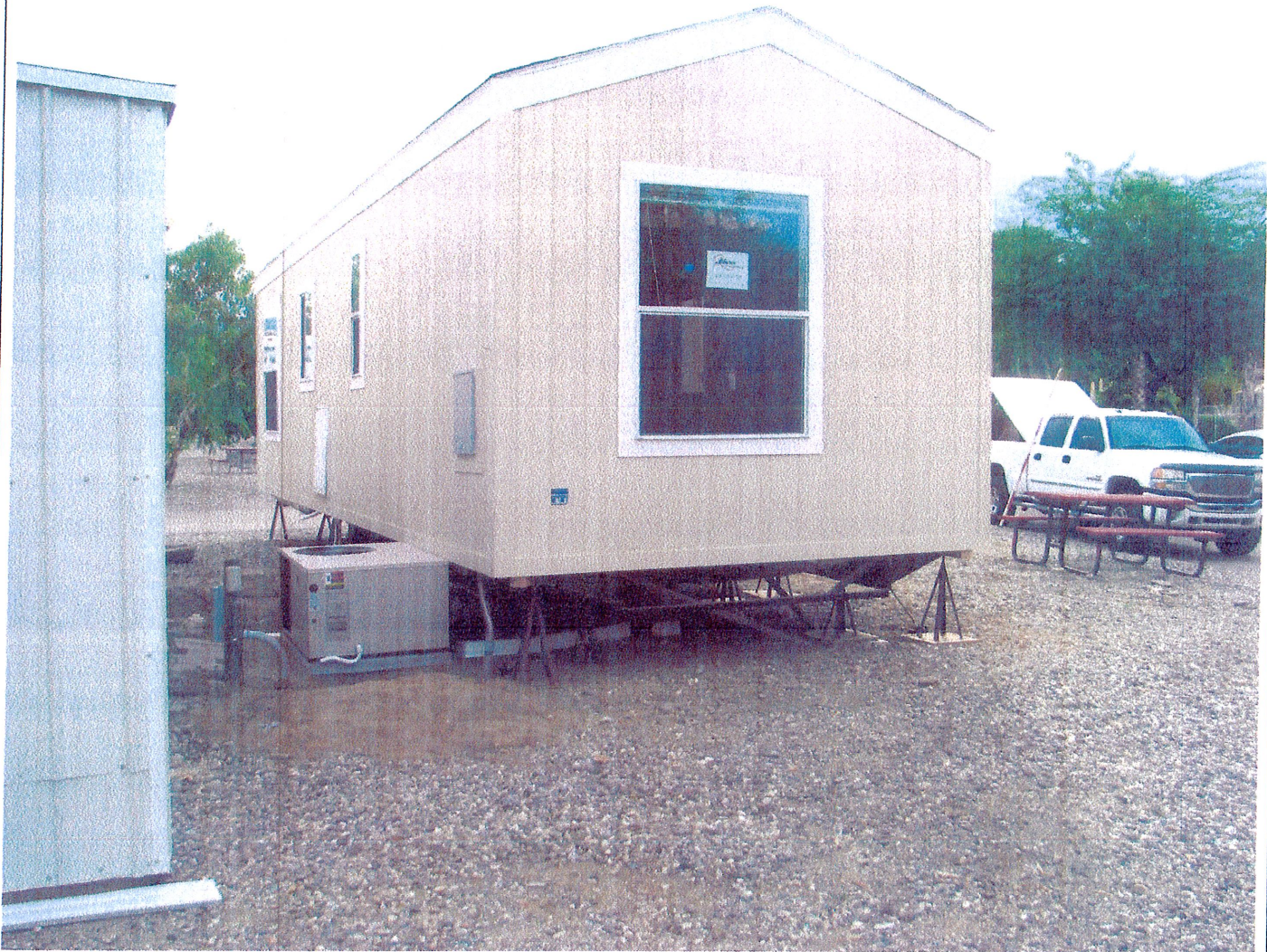
WEST END/NORTH SIDE. C2E ON A/C PAD (PHOTO 10-22-14)
