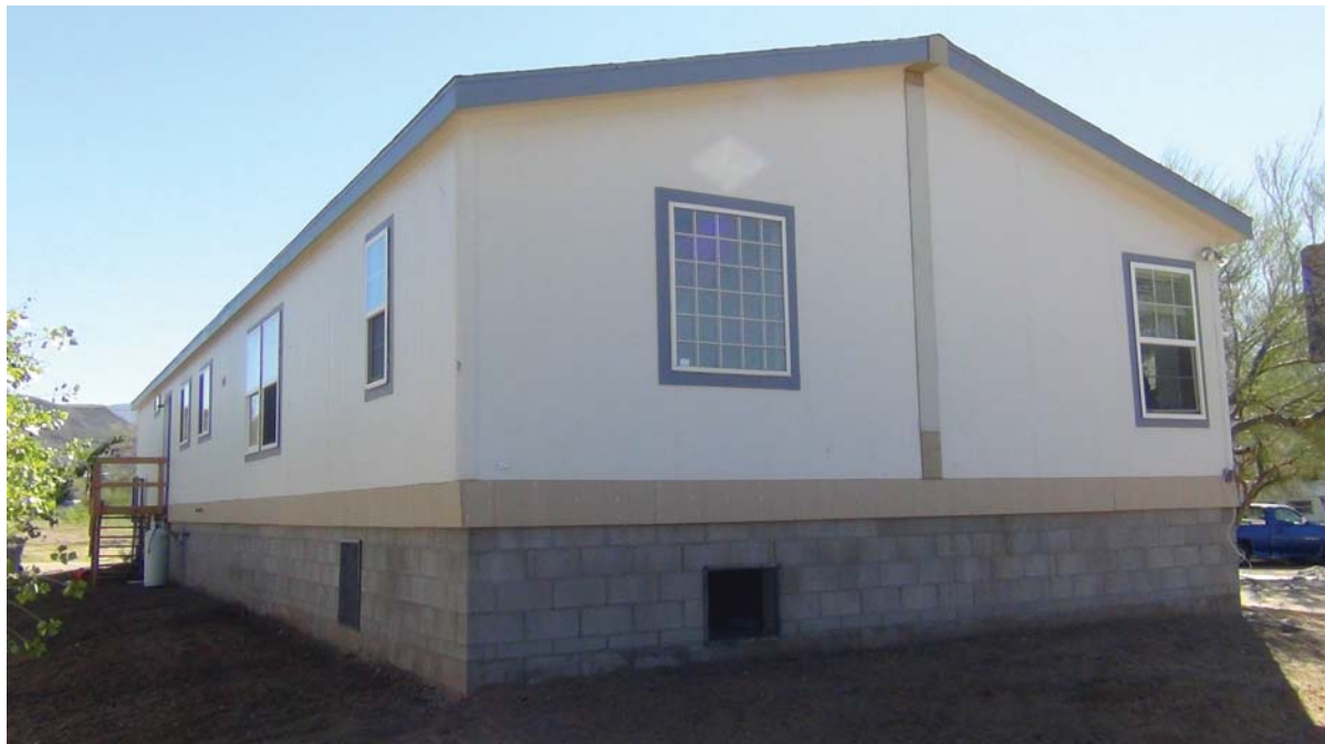
REAR OF HOME, FROM LEFT REAR CORNER
